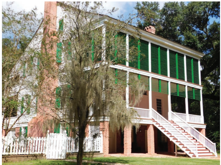
ABOVE: The house, restored in the late Federal Period style, and its grounds have been part of the Audubon State Historic Site since 1956.
